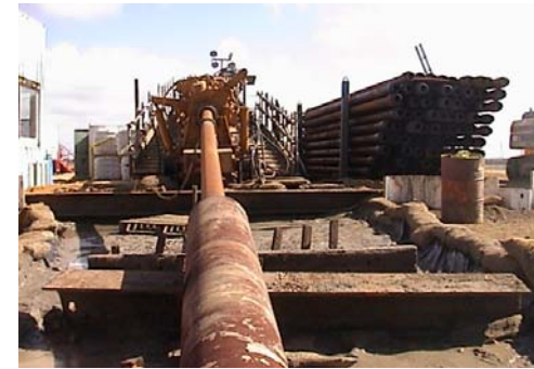
COEDRILL 550 Pilot Hole Operation
