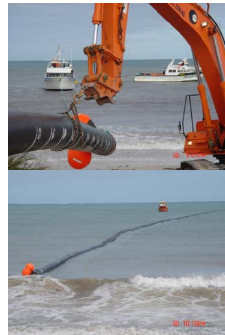
28" HDPE Liner Tow Out Operation
