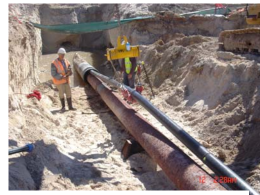
10" Concrete Coated Production & Umbilical Conduit Installation in 28" HDPE Liner.
