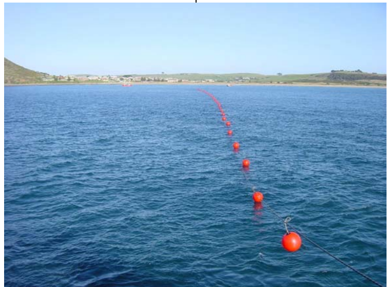
Below: Cable Line at Stanley, Tas
