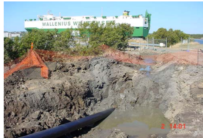
Top: Pipeline Installation Operations at Yarra Street Pinkenba.
