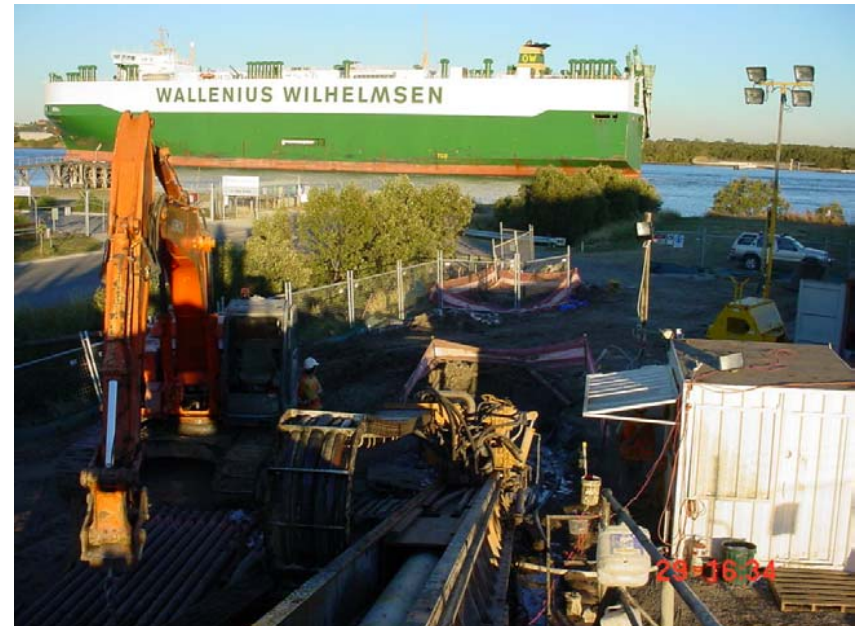
Top: Drilling Operations at Yarra Street Pinkenba.
