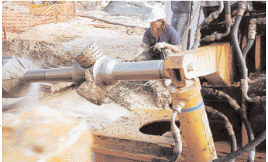
Above: Completion of 30" rock reaming on the Tweed River.
