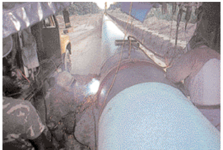
Above: Welding of the "McDow" coupling.
